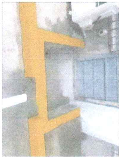
EXIT DOOR ENCLOSURE 2 FLOOR DRAIN WITH 4" PVC DRAIN PIPE TO EXISTING DRAINAGE
